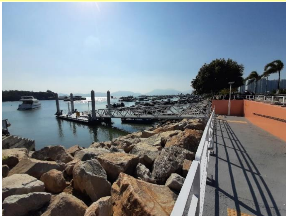
Example: Floating pontoon at Tuen Mun Area 27
